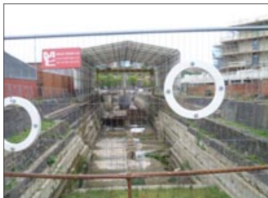
▲ The dry dock is still in use.
