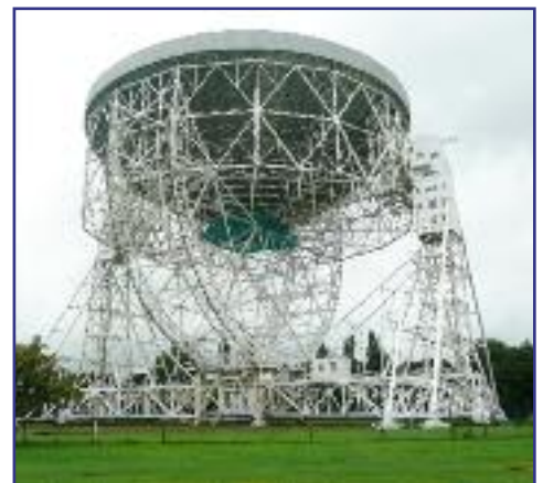
▲ The Lovell telescope was built at enormous expense and came in well over budget! Completed in 1957 and measuring 76.2m in diameter it replaced the 1947 Transit Telescope to become the largest fully steerable telescope in the world.
