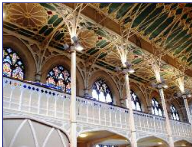
▲ The interior of St George's is a complete surprise with slender iron columns and a beautiful structural latticework bathed in light. Cast iron rafters support modular painted slate
