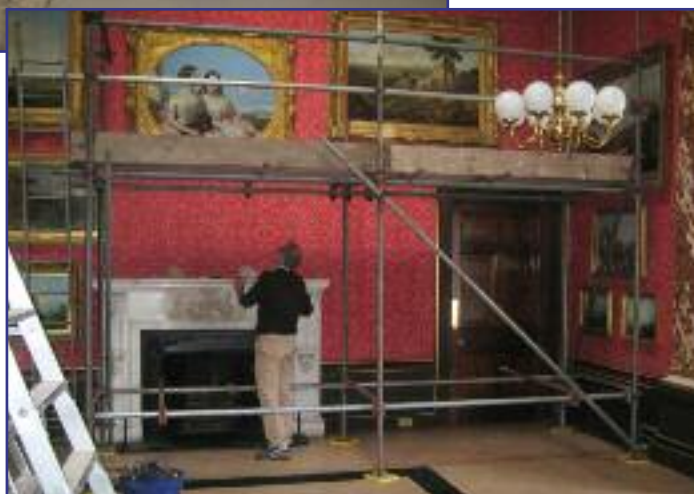
▶ David Lippiatt overseeing the removal of paintings from the Blaise Picture Room following a water leak caused by heavy rain
