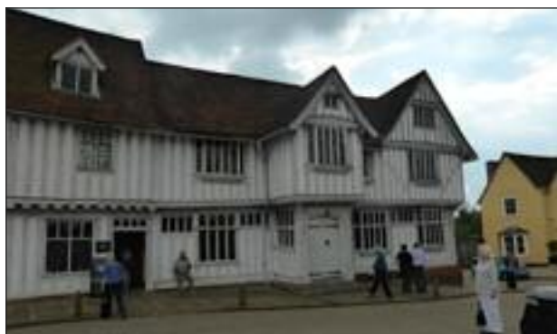
▲ Clothier's houses had wicket doors like this one – a small personal door set into a much larger one - which allowed the wool to be brought into the building on the packhorses.
