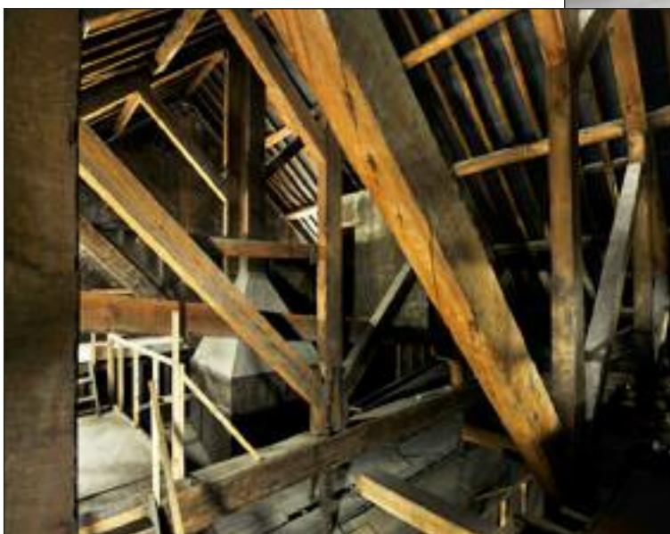
◀ Georgian roofspace – containing the unique 'Thunder run'
