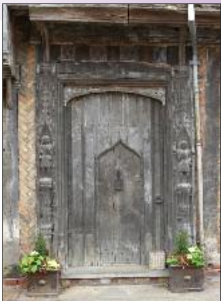
▲ Clothier's houses had wicket doors like this one – a small personal door set into a much larger one - which allowed the wool to be brought into the building on the packhorses.
