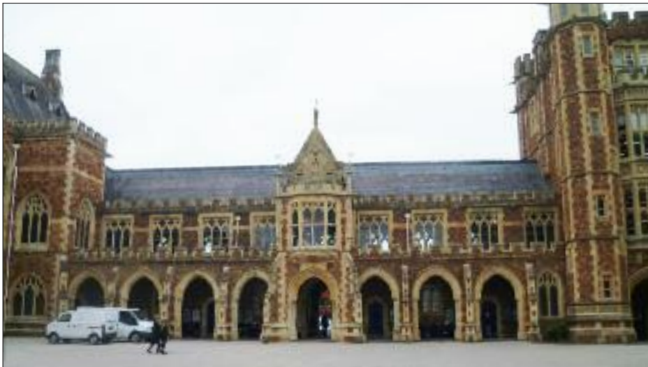
▲ Senior school buildings Photo by Catherine Dixon
