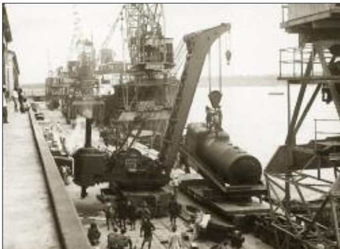
◀ Unloading a locomotive boiler at Kilindini harbour, Bombasa, Kenya Image from the BECM image collection ©BMGA
