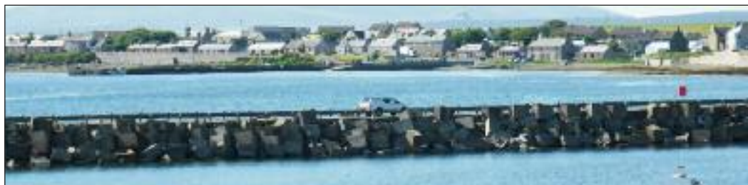
◀ The Churchill Barriers were made from 66,000 locally cast 5- and 10-ton concrete blocks
