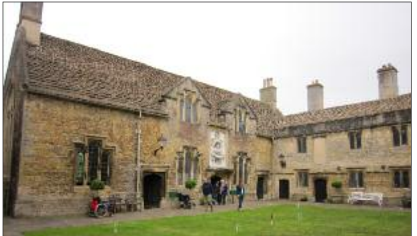
▲ Sexey's Hospital showing the oldest part of the quadrangle 1638. Hugh Sexey had died in 1619 and the Trustees built a 'hospitium' to house the poor - it continues today as a charitable institution to house 25 residents with a Bruton connection
