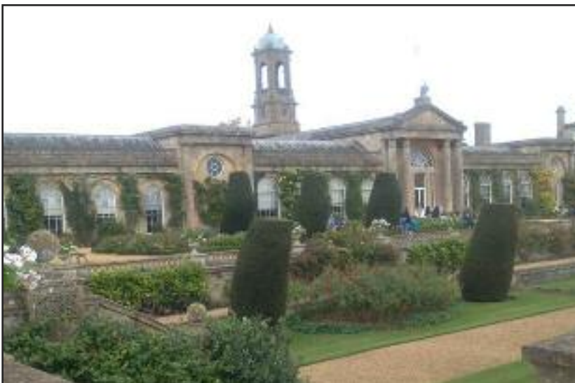
◀ Bowood House showing part of the formal garden
