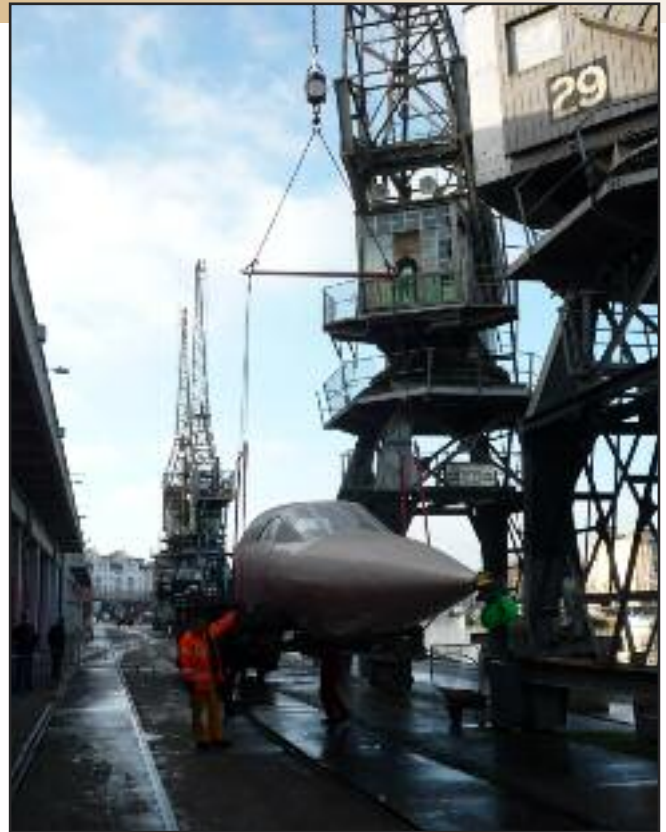
▲ Crane 29 lifting the Concorde cockpit onto its new trailer Photo © Chris Ecclestone
