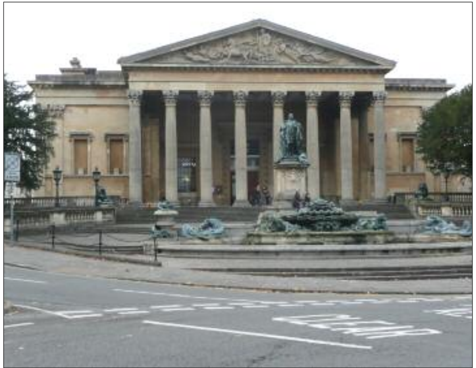
▲ The Victoria Rooms on Thursday 3 November 2016
