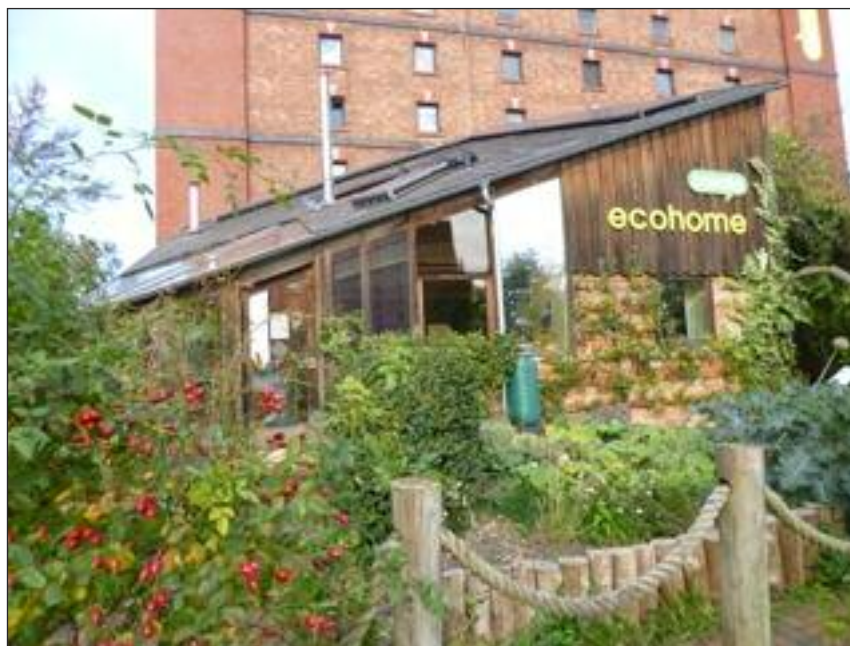
▲ The Create Centre and the Ecohome
