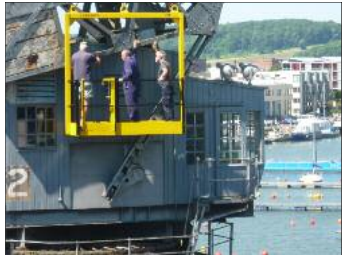
▲ Painting the cab of M Shed Crane 29
