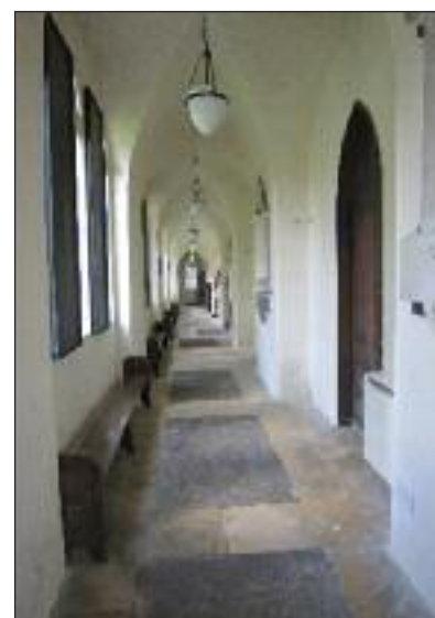
▲ St Mary's Church Tetbury showing the North Ambulatory which is a corridor giving the only access to the side pews
