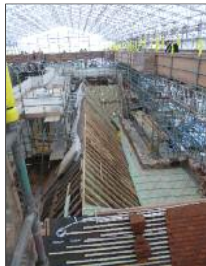
▼ Fine craftsmen repairing the roof Photo Carol Ouvry
