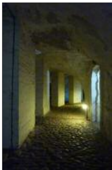
▲ There was a labyrinth of cellars and store rooms under the castle
