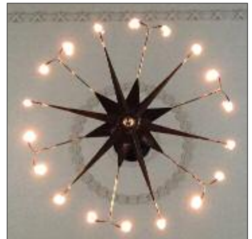
▼ The great courtroom gasolier, with 18 open-flame burners blazing
