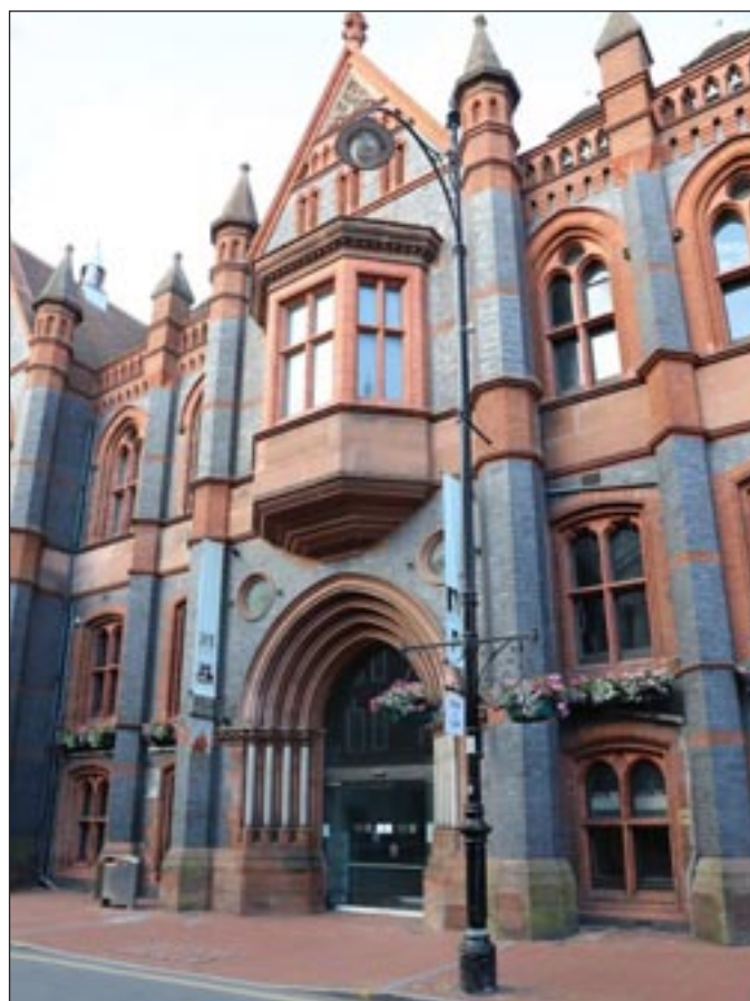
▼ Reading Museum is housed in the Town Hall
