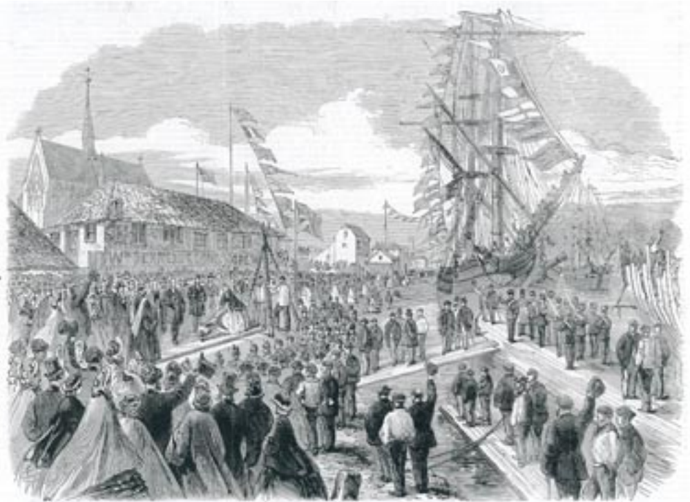
▲ Princes Wharf, 1863: Laying the first rail of the line that was never completed © Bristol Culture
