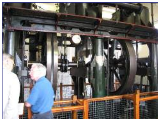
▲ The vertical inverted triple expansion steam engine was installed in 1895 and is still running.
