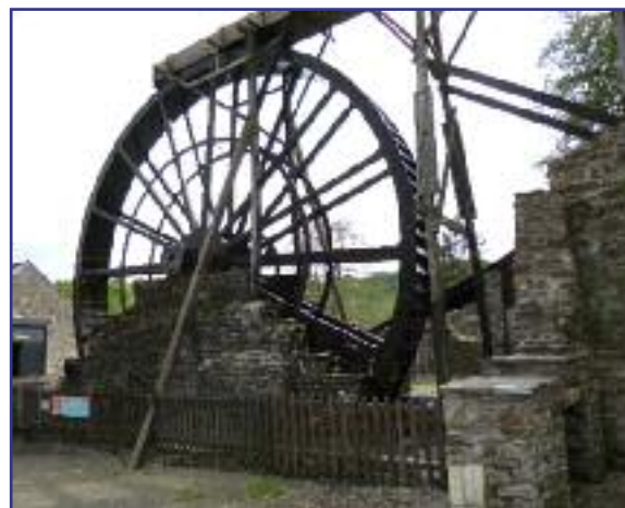
▲ The overshoot waterwheel turned sedately providing green power for the quay.
