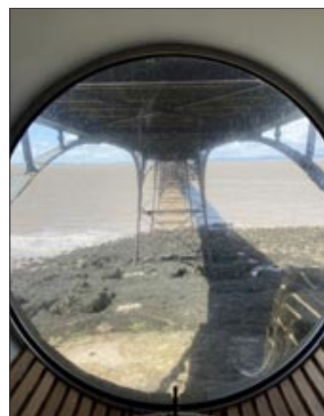
▲ Porthole view of the structure of Clevedon Pier
